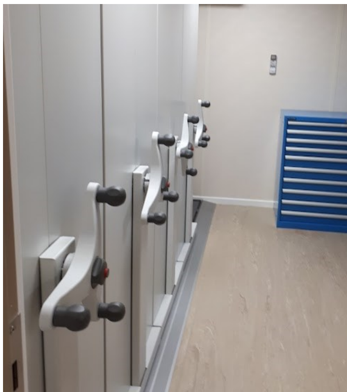
Visitors are fascinated by the modern roller racking installed to store and protect our precious archives.
